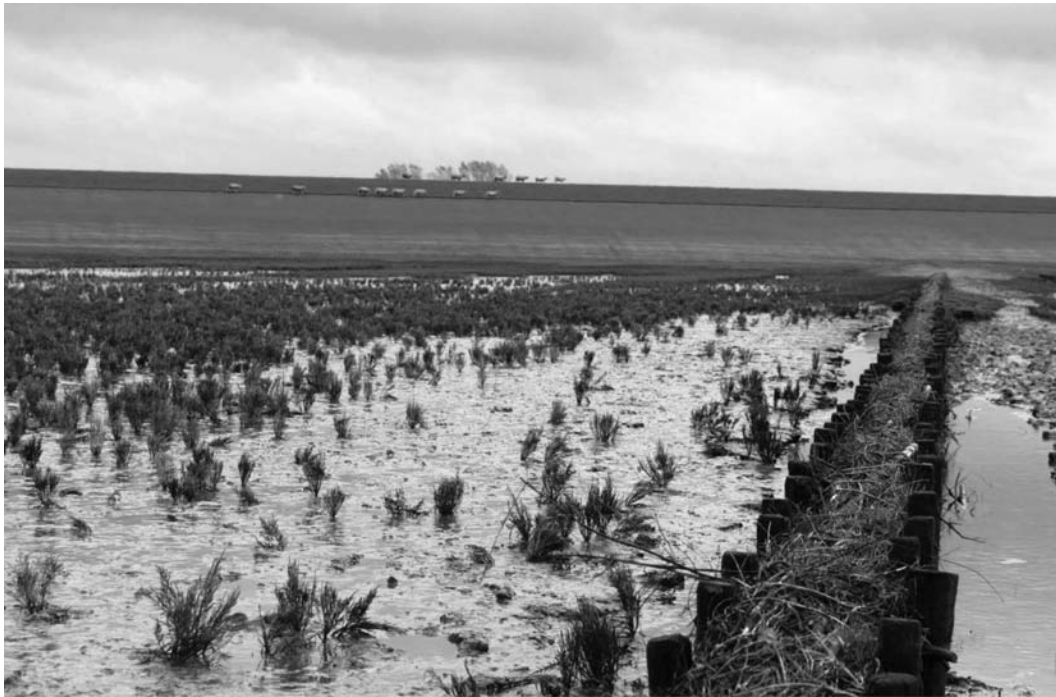
Figure 8.8 Brushwood dams to create artificial sheltering of salt marsh vegetation against waves and currents. (Photo courtesy of Vincent Vuik.)
